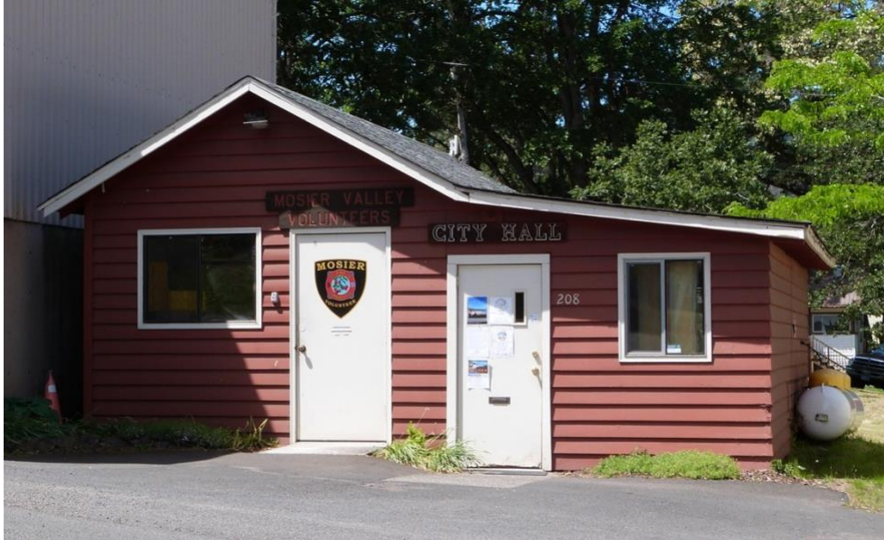
Existing Mosier Fire District Office (door at left) and Mosier City Hall (door at right)
